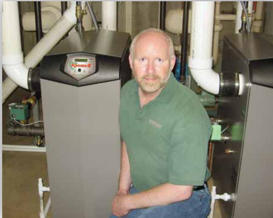
Don Smet, Designer Standard Plumbing Heating Controls Corp., Spokane, WA
